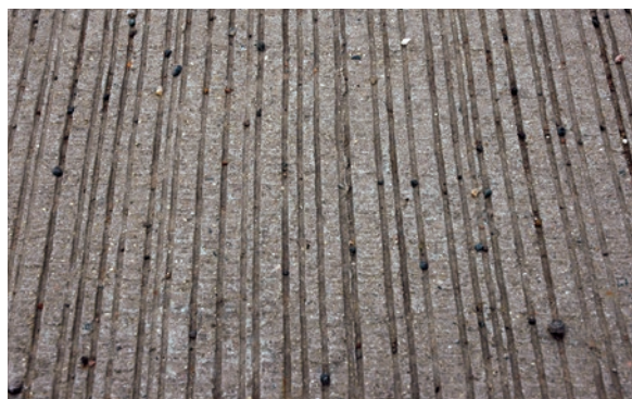
Figure 1.16 Typical hessian-drag and tined finish
