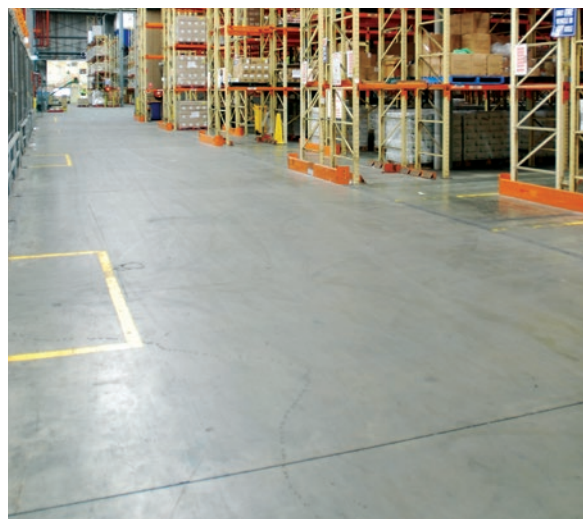
Figure 1.12 The designer should give careful attention to the joint layout
