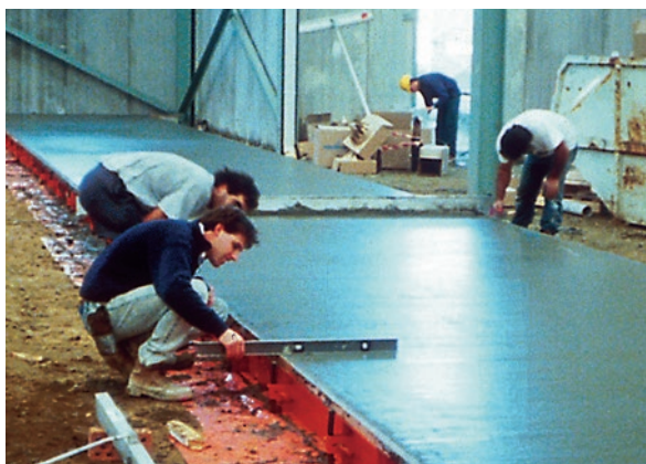
Figure 2.21 Ensure concrete is kept level with side forms
