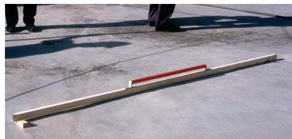
Figure 2.34 3-m straightedge used to assess surface tolerance
