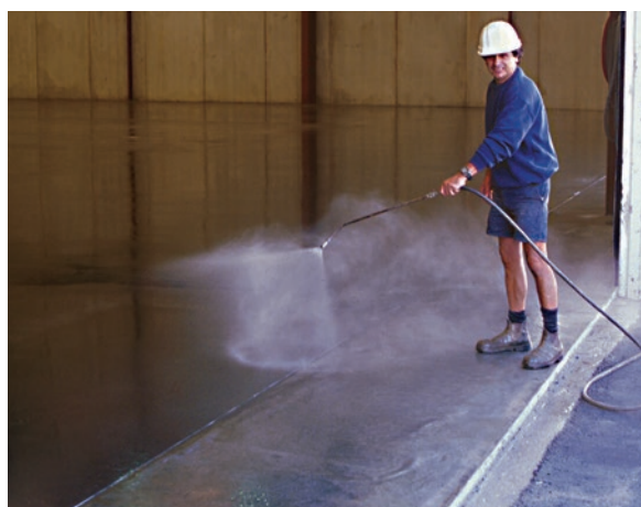
Figure 2.28 Liquid membrane-forming curing compound being applied by spray
