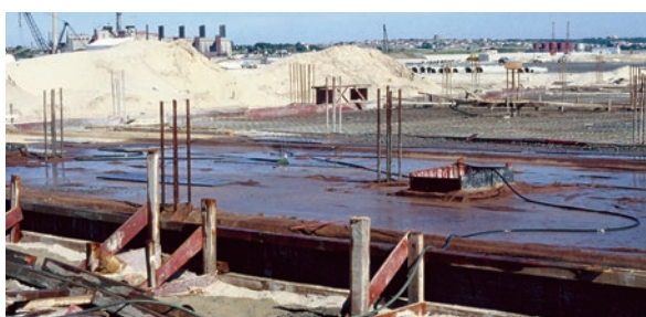
Figure 2.25 Ponding and covering with hessian
