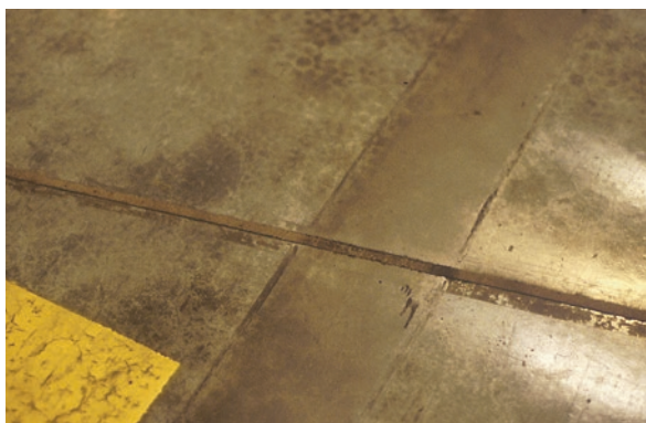
Figure 1.6 Epoxy filling of contraction joint
