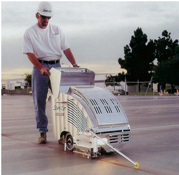
Figure 2.30 Early-entry saw being used to cut sawn joint
