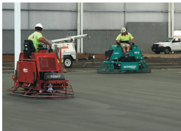
Figure 2.23 Double and triple-head power trowel machines are now commonly used in Australia for major warehouse projects
