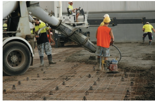
Figure 2.6 Reinforcement chairs provided as work proceeds
