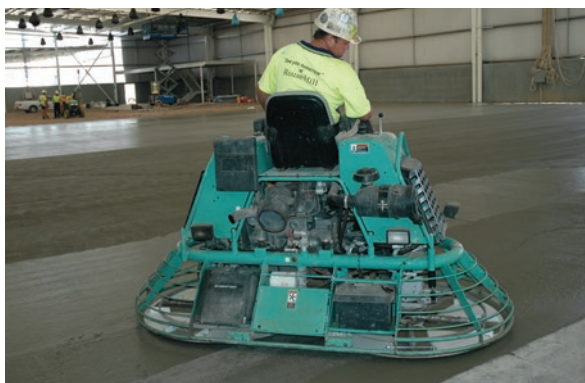
Figure 2.19 Base surface being power floated
