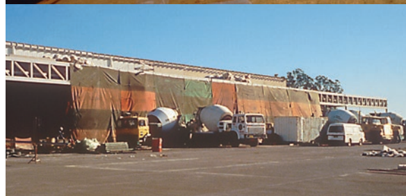
Figure 2.24 Examples of wind breaks to protect concrete from rapid drying
