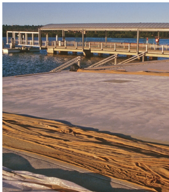
Figure 2.26 Wet hessian used for curing
