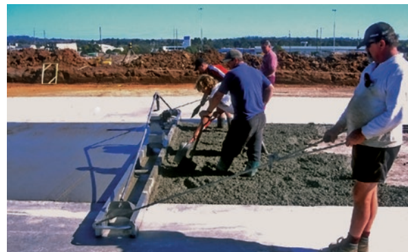
Figure 2.13 Base being compacted with a double vibrating beam
