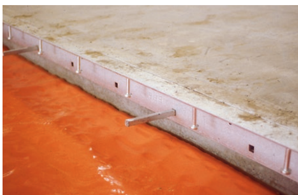
Figure 1.7 Armouring of joint edges with steel angles
