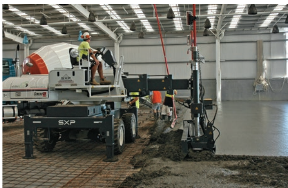
Figure 2.16 Pavement surface being compacted and levelled with a laser screed
