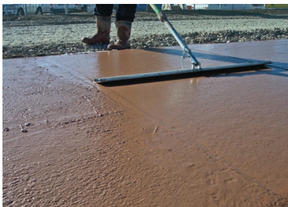
Figure 2.17 Initial floating of pavement surface with a 'bull' float
