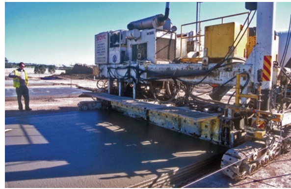
Figure 2.9 Slipform paving of industrial floors and pavement
