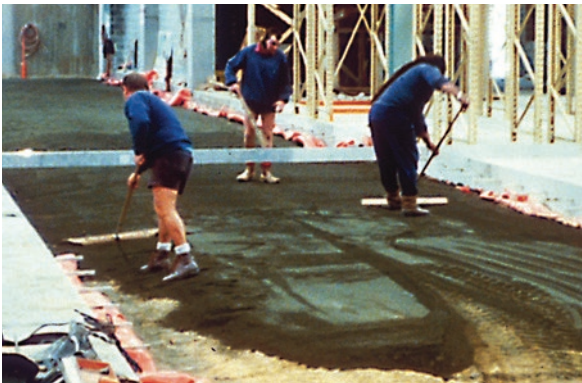
Figure 2.4 Subbase level checked using a straight edge and timber gauge.
