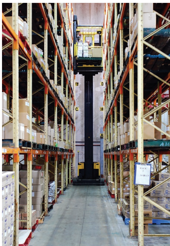
Figure 1.17 Typical storage facility with narrow aisles and high racks in which floor flatness is critical
